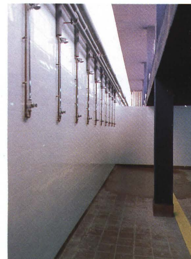
Interior vestuarios. Interior of locker room.
