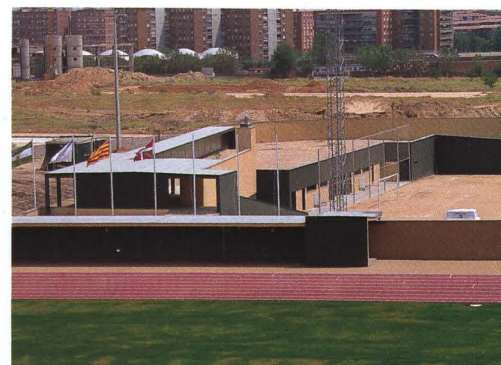
Vestuarios. Locker rooms.
